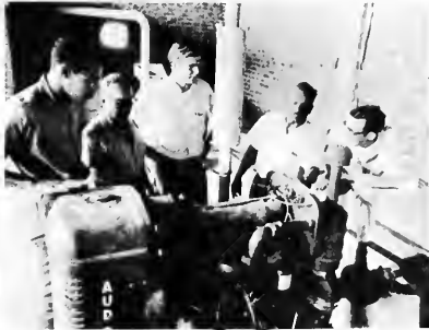
Peace Corps volunteers Jim Hairston (left) and Hank Coleman (right) discuss the installation of a new power unit at a rice mill in Tumbes, Peru.
